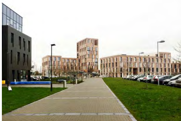
Figure 14.10 - Courtyard Student Apartments (Source: Maynooth University)
